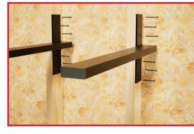
2. Place brackets between 16-20 inches apart, or where wall studs are available. Using the bracket holes as guides, drill pilot holes into your wall studs. After pilot holes have been made, fasten your brackets to the studs with screws. Ensure, brackets are level.
