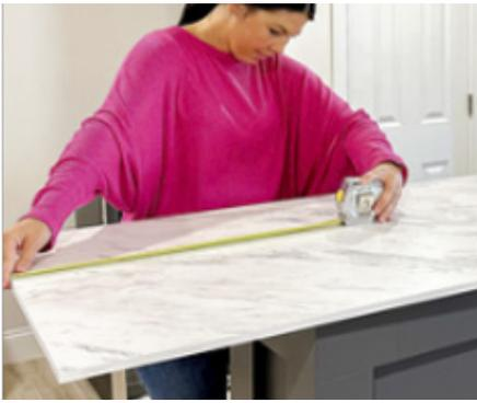
**PART 1** Measure the top and compare measurements to the cabinet. Provide minimum 1/8 in. gap at all walls.
