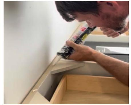
**PART 3** Secured top with 100% Silicone Adhesive sealant every 12 in. - 18 in. along the back of cabinet supports. Apply an 1/8 in. (3.2MM) lineal bead along the entire front cabinet frame length.
