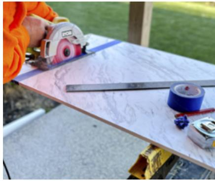
**PART 2** Cut composite countertop to length with carbide saw blade. Use painters' tape to protect surface from abrasion. Lightly sand edges if needed.
