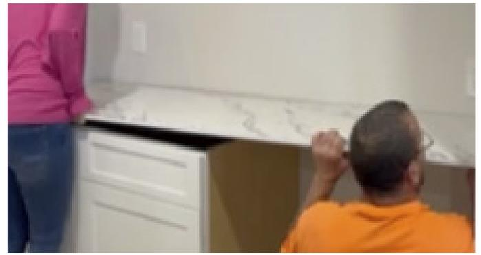
**PART 5** Position countertop in place. Press down firmly on countertop and make sure top is level. Facing overhang should be approximately 1 in.
