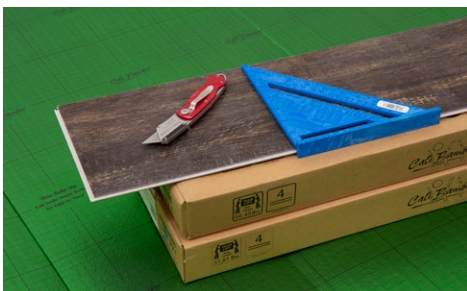
Cutting boards using Score and Snap technique
