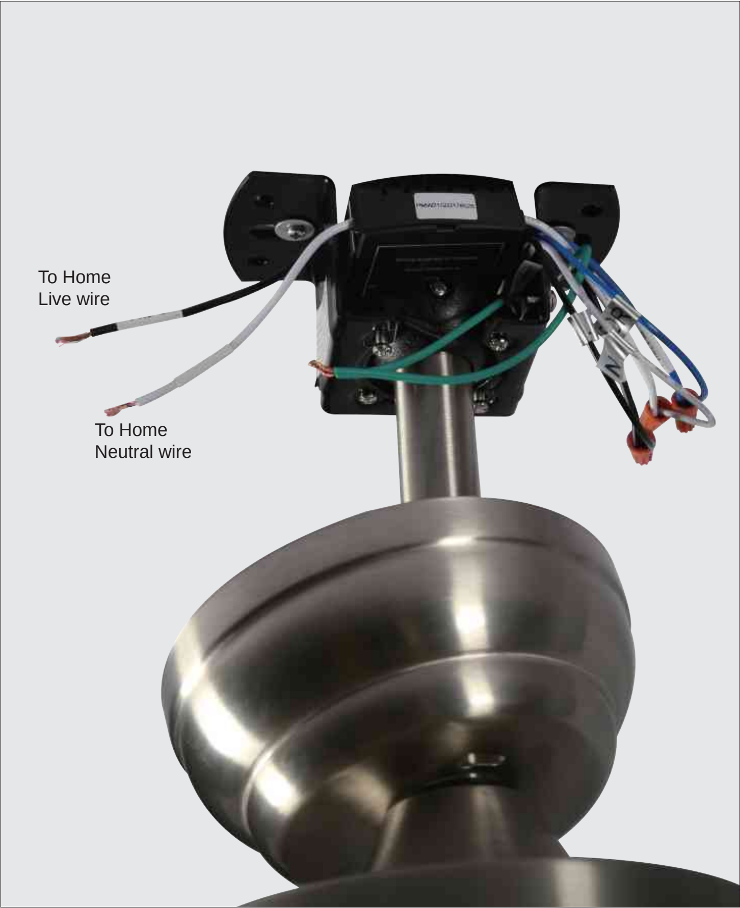
Step 13 Connect the receiver to home wires. Black for Live wire, White for neutral wire, Green for ground wire.
