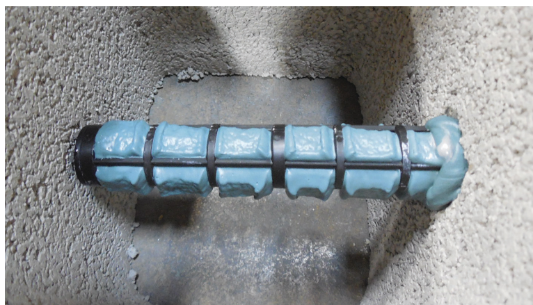
Hollow CMU Install with Opti-Mesh Screen
