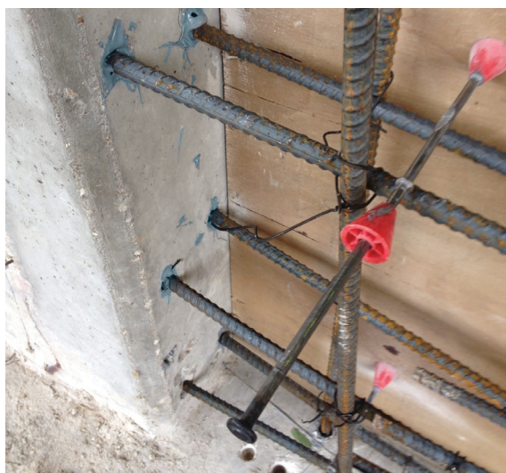
Rebar Wall Extension
