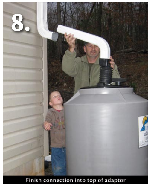
Secure all connections & seal with silicone.
