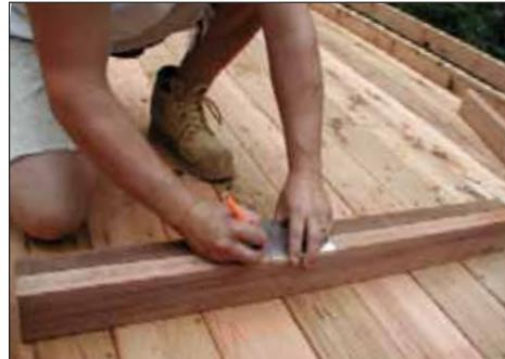
**Step 3:** Screw on Deckorators Estate baluster connectors (sold separately) on each mark.
