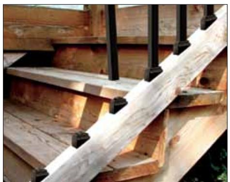
**Step 4:** Place the bottom rail (2x4) on 3" blocks (2x4 scrap material works best) and attach to the post. For easy rail-to-post connection, we recommend using Deckorators railing connectors (sold separately). Put clear adhesive on each connector to properly secure balusters and prevent spinning. Insert balusters over baluster connectors.
