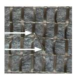
FibaLath should be installed with a minimum 3" overlap across seams.
