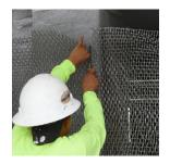
Attach FibaLath with recommended fasteners depending on framing structure.
