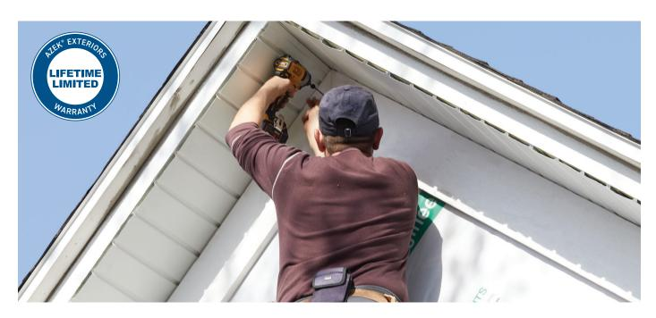
AZEK's lightweight and durable trim made from engineered polymer and lasts longer than wood but can be cut, drilled and fastened with standard woodworking tools. **See inside to learn key installation differences and best practices.**
