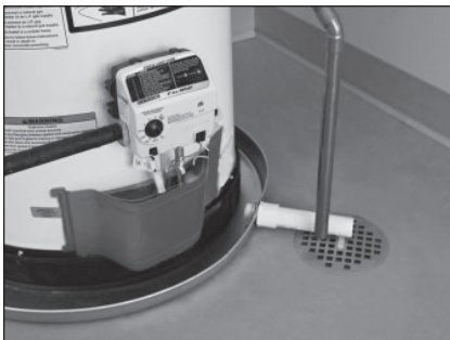
Figure 23 - Metal drain pan piped to drain.
