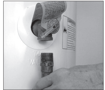
Figure 21 - Removing the T&P Relief Valve discharge pipe.
