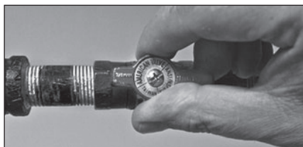
Figure 33 - Gas valve in "on" position
