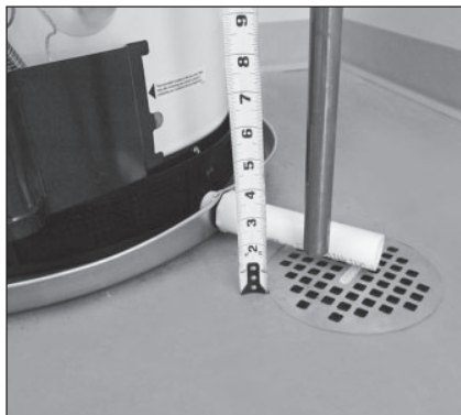
Figure 26 - Temperature and Pressure Relief Valve Pipe
