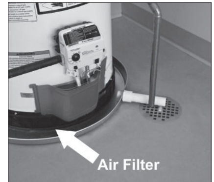
Figure 24 - Filter attached to water heater.
