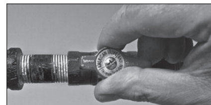
Figure 51 - Gas valve in "on" position.
