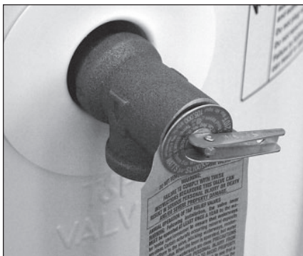
Figure 25 - Temperature and Pressure Relief Valve
