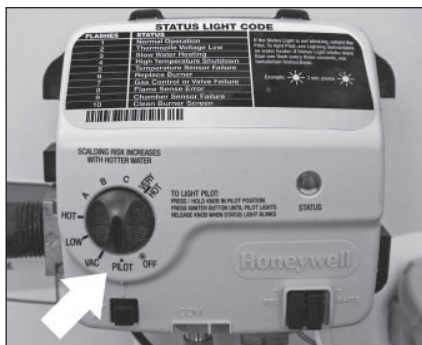
Figure 34 - Gas control/valve.
