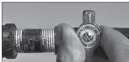
Figure 47 - Gas valve in "off" position.
