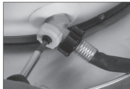
Figure 20 - Draining the old water heater.
