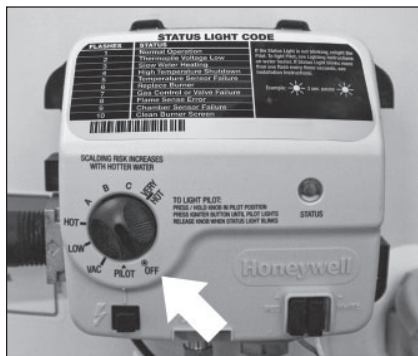
Figure 46 - Gas control valve.
