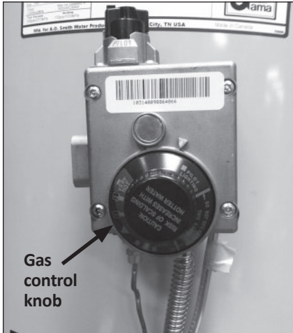
Figure 17 - Turn gas control/temperature knob OFF.
