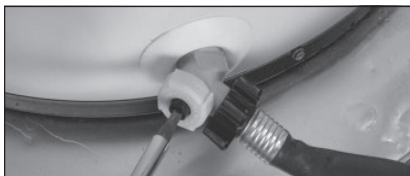
Figure 41 - Draining the water heater.
